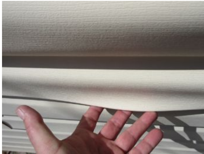
Damaged siding
