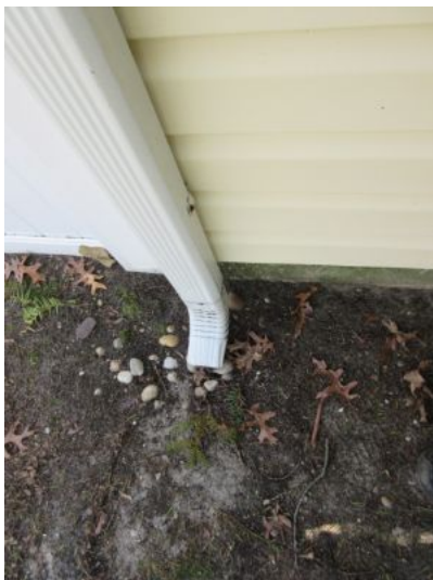
Install splash blocks
