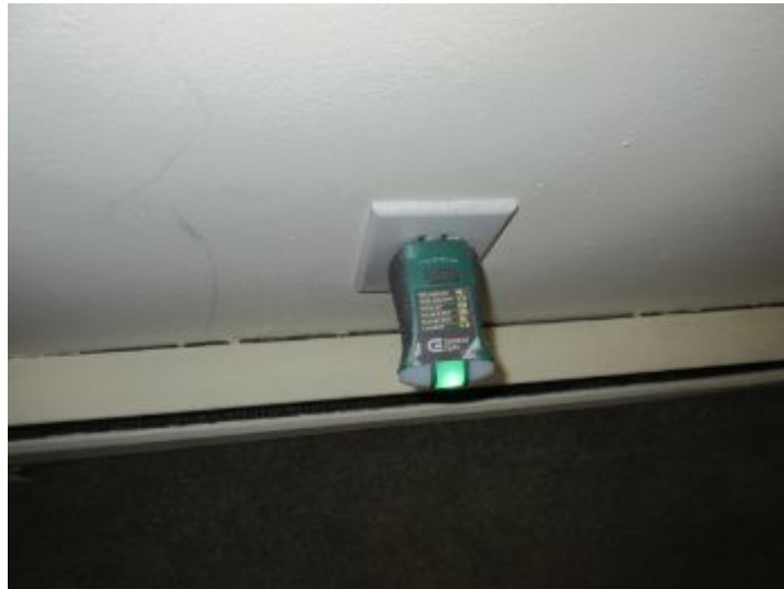
Interior Areas and Rooms Receptacles
