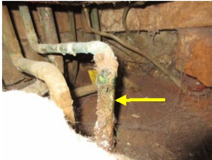
Pipe deterioration
