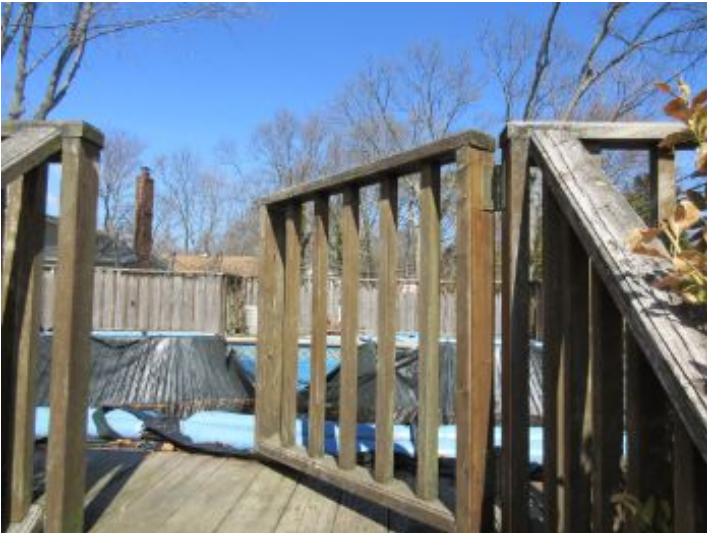
Pool deck gate
