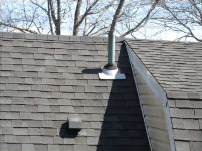
Roof Vents and Hood Penetrations
