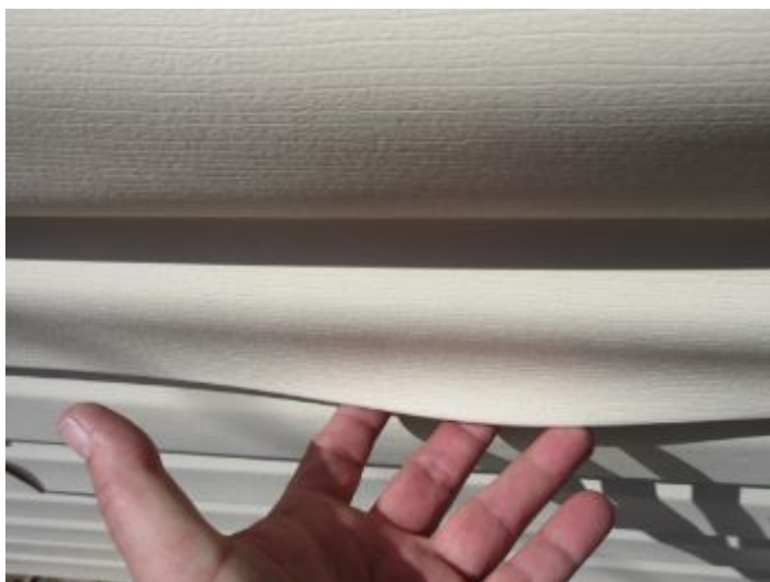
Damaged siding
