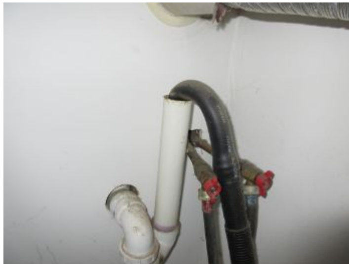
Laundry Washer Connections & Drain
