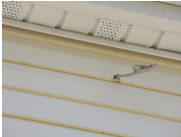
Missing light fixture
