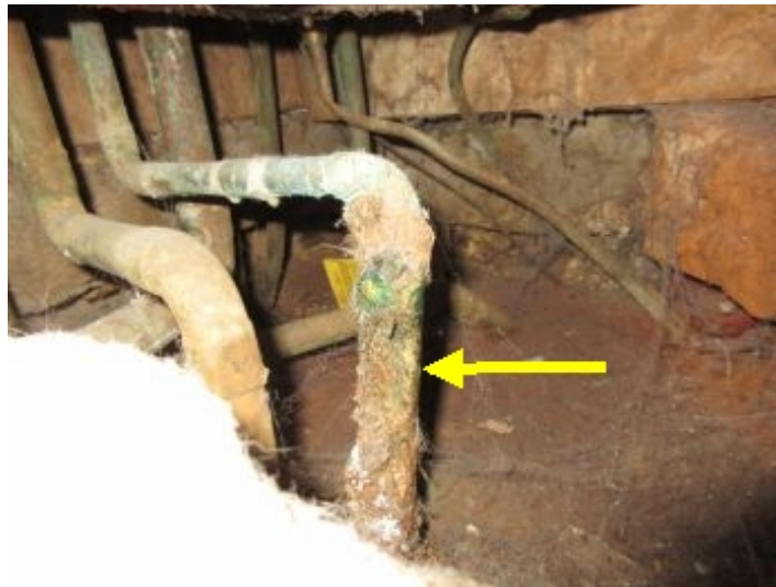
Pipe deterioration
