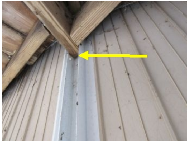
Addition support needed
