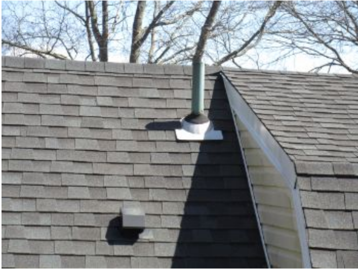
Roof Vents and Hood Penetrations
