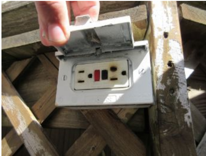
Damaged pool side GFCI
